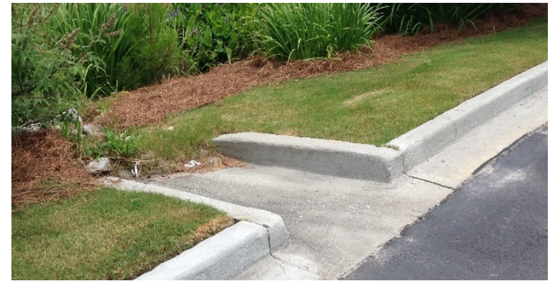
Figure 4.08.2. Concrete Curb with Drainage Opening
